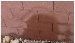
Water soaking through a wall from a missing drip head on the <u>opposite</u> side of the wall for a long period of time.
