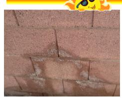
Efflorescence caused by water soaking through a wall from a missing drip head on the opposite side of the wall for a long period of time.
